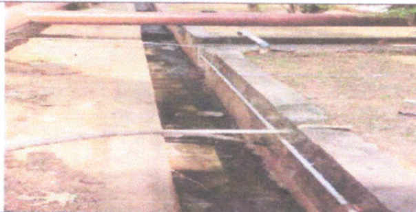
One more drain effluent stagnated (effluent from the STP out let utilized for gardening (seepage from the back of the treatment facility area )
