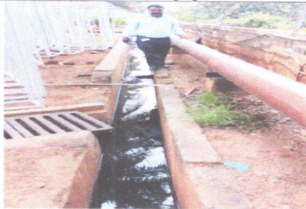
Discharging the vehicle wash water to storm water drain
